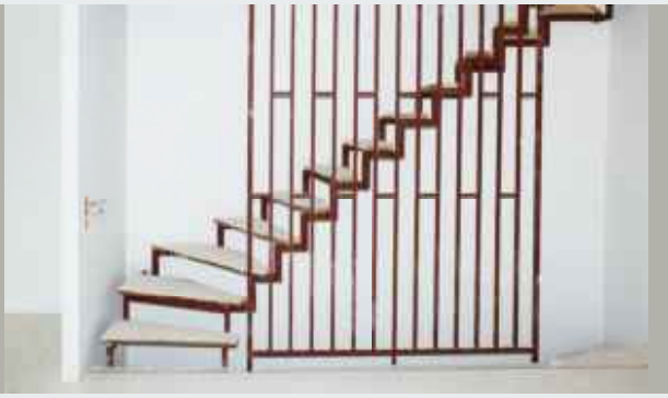
Decoupled harp staircase as skeleton structure
