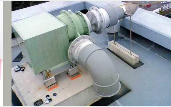
Point bearings for a air handling unit
