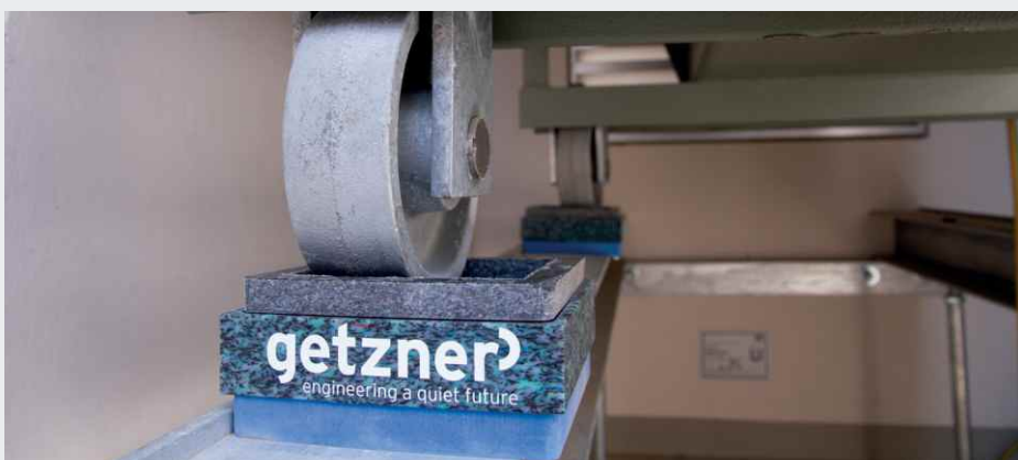
Vibration decoupled bearing of a distribution transformer with TR transformer pads
