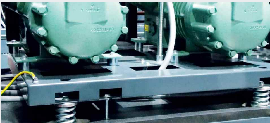
Bearing of compressors using Isotop® SD steel springs
