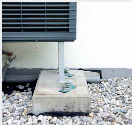
Bearing of an outdoor unit on the floor (foundation) using Isotop® MSN elements
