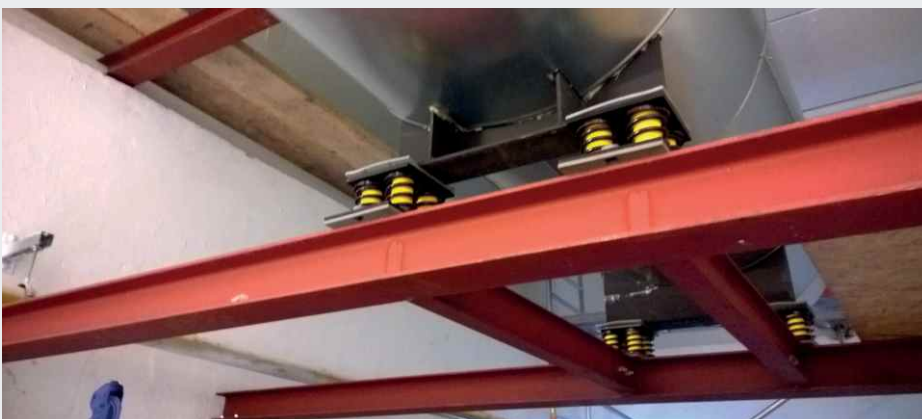
Bearing of an exhaust heat exchanger using Isotop® DSD-BL
