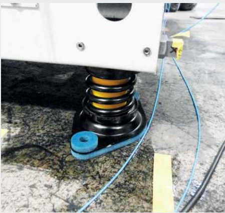
Bearing of an industrial heat pump using Isotop® DSD and FP/K footplate with damping element
