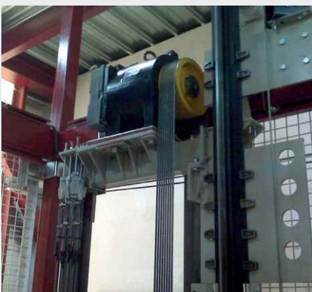
Decoupling of the drive using pre-stressed bearings made from Sylomer®
