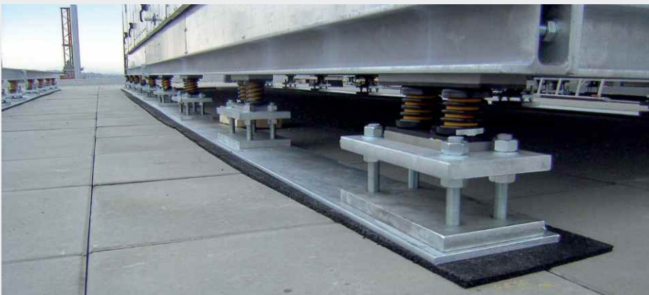
Low-frequency bearing of an AHU on steel springs with an integrated damping core (Isotop® DSD-BL)
