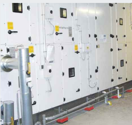
AC system next to office space decoupled with Isotop® SE
