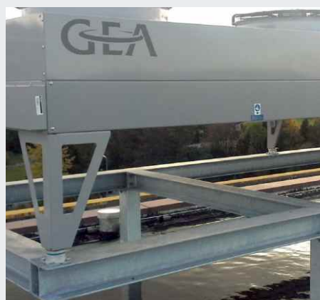
Structurally-strong bearing of a cooling tower using Isotop® DZE
