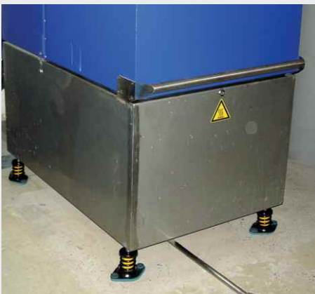
Small combined heat and power plant decoupled with Isotop® DSD and FP/K footplate
