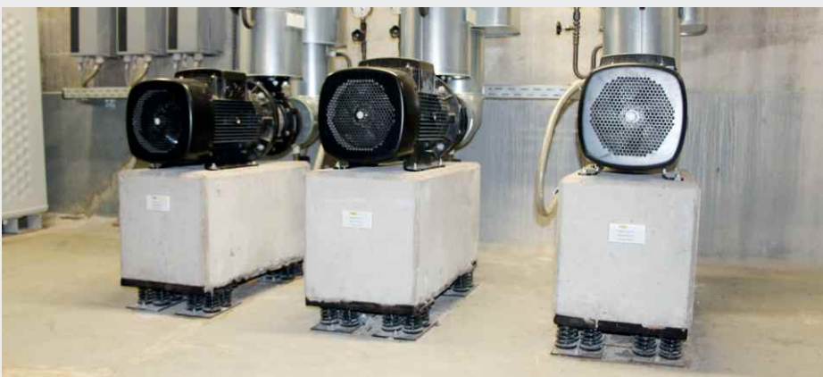
Pump bearing with additional mass (foundation) on Isotop® SD block elements
