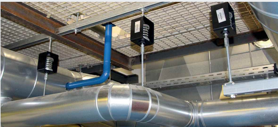
Pipes decoupled using Isotop® SD/Z
