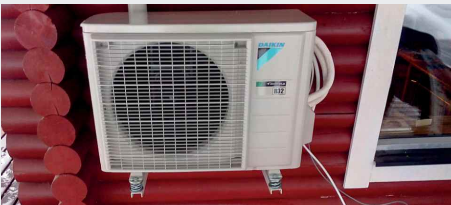
Bearing of a suspended outdoor unit using Isotop® MSN elements
